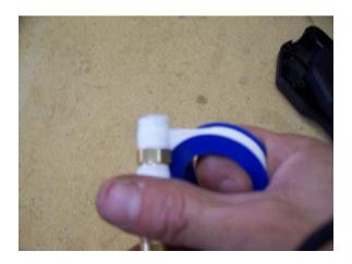
2) Install the valve assembly to the shut off valve until hand tight, then grasp it firmly with a pair of channel lock pliers and use a 9/16" wrench to tighten to appropriate angle. It may be necessary to hold the valve up next to the handle of your 360 to insure proper installation angle.
